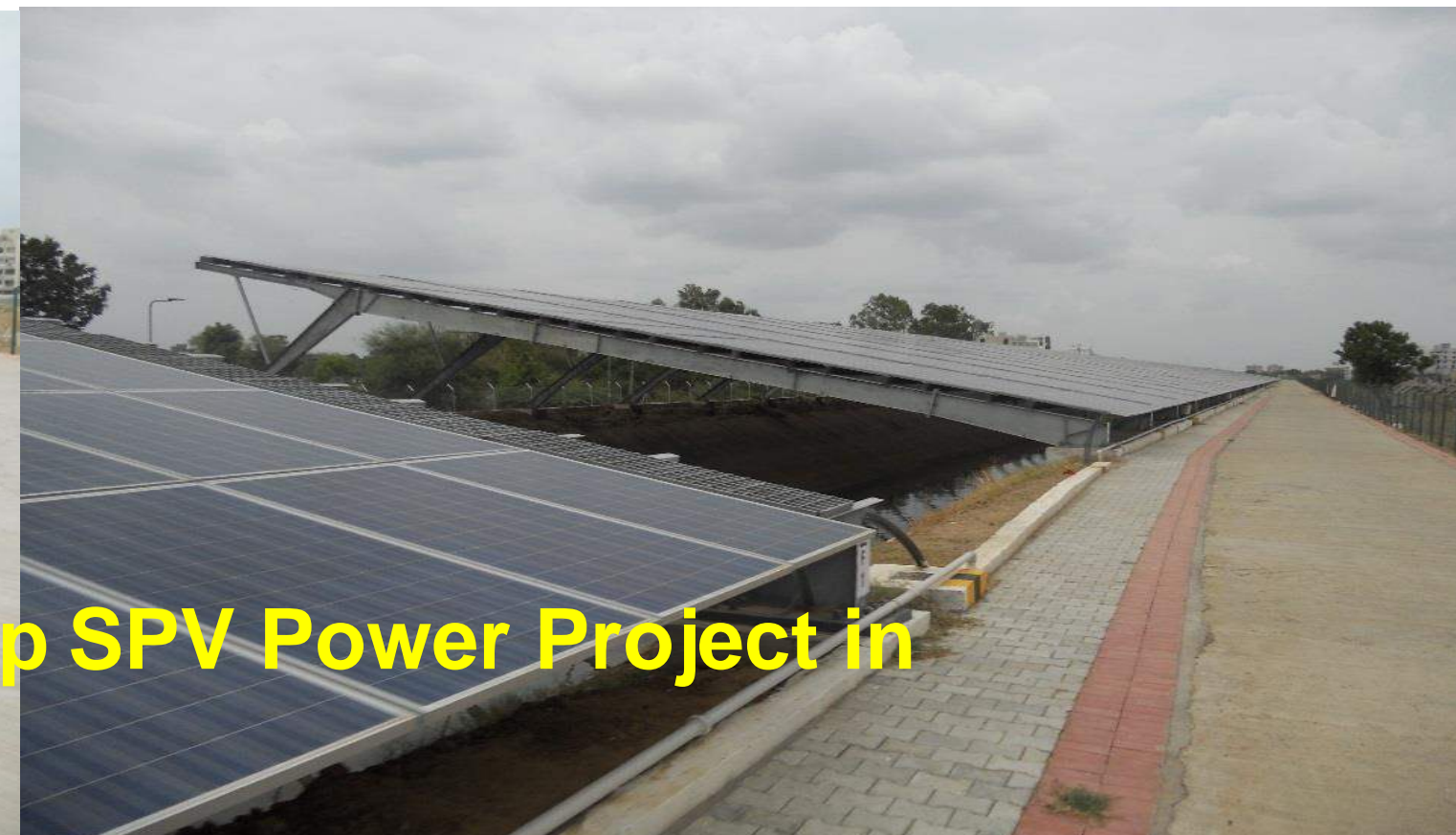
1 MW Canal Top SPV Power Project in Karnataka
